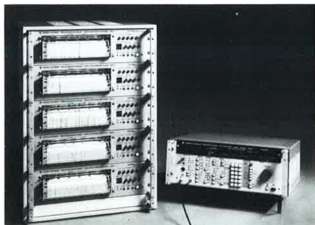
radiomonitoring/recording system. Recording is electrosensitive, producing a black trace at the point where the recording electrode touches the paper when the electrode voltage is applied. This so-called Z control is accomplished by the processed signal of the receiver output.
